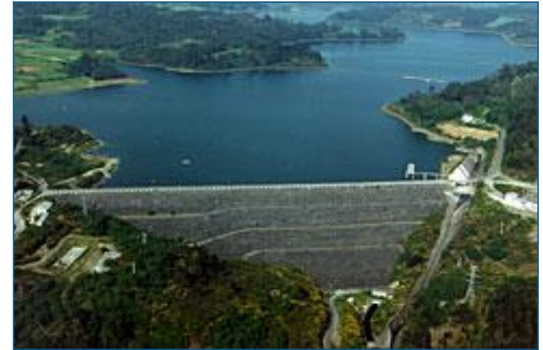
Portomouros hydroelectric dam.
